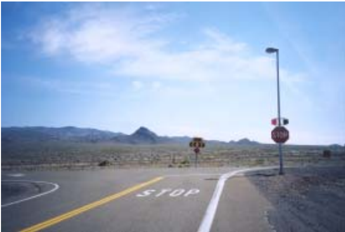
Flashing beacon at the intersection of U.S. 95 and U.S. 6 in Esmeralda County.
