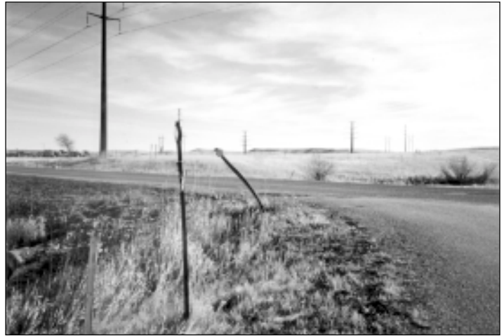
Examples of a bent stop sign support and bent and damaged delineators.
