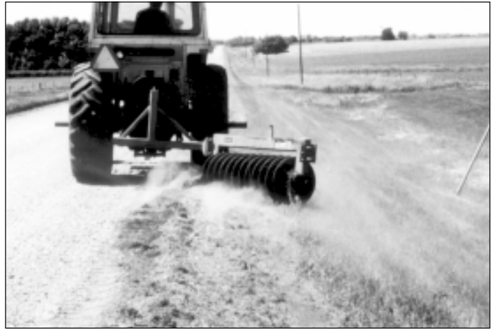
Mulching a gravel road shoulder with a shouldering disk.
