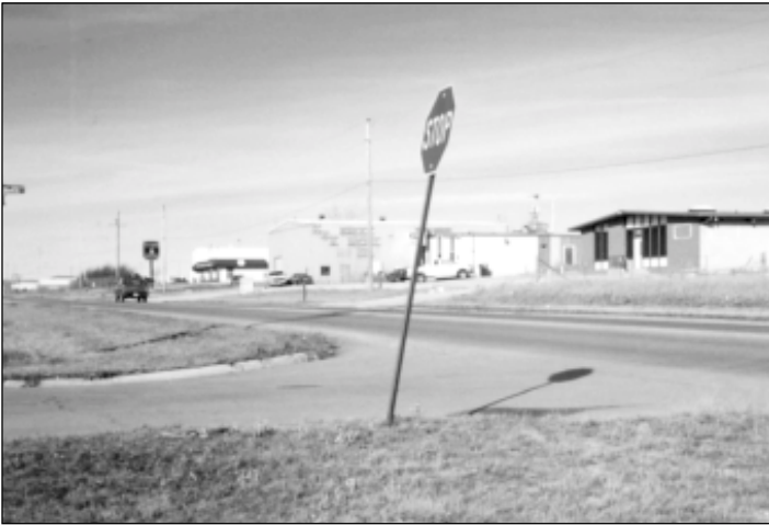
Examples of a bent stop sign support and bent and damaged delineators.
