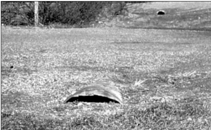
The silting and debris in these culverts need attention before spring and summer rains begin.
