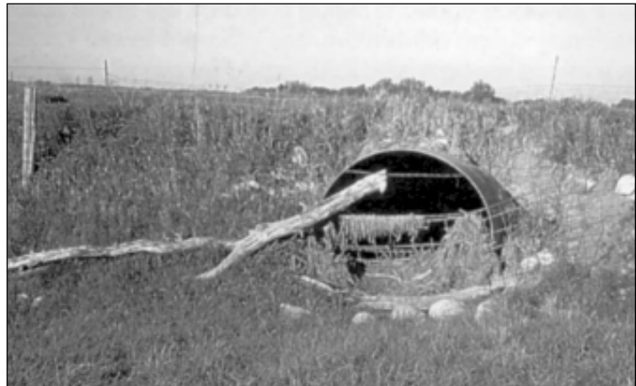
The silting and debris in these culverts need attention before spring and summer rains begin.
